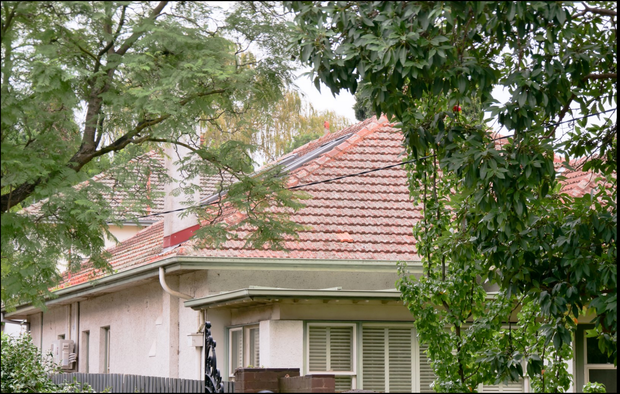
Only skylights are visible from the street
