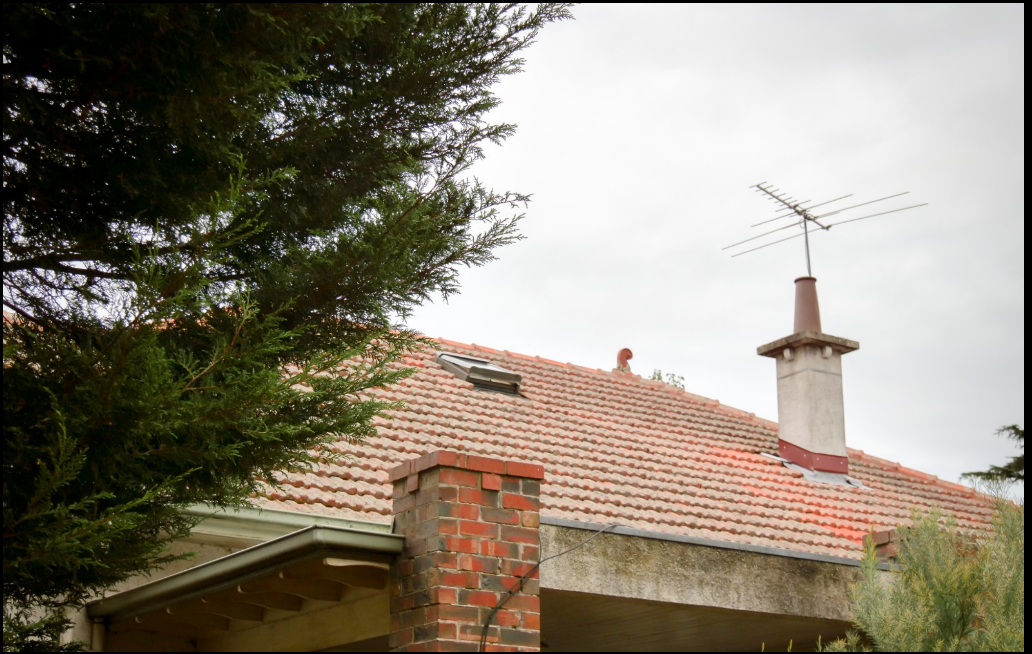
Only skylights are visible from the street
